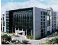
Taoyuan Technology Center (Green Building)
